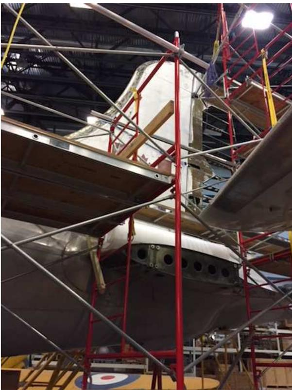
*Scaffold erected next to North Star to support removal of the rudder and vertical stabilizer.*
